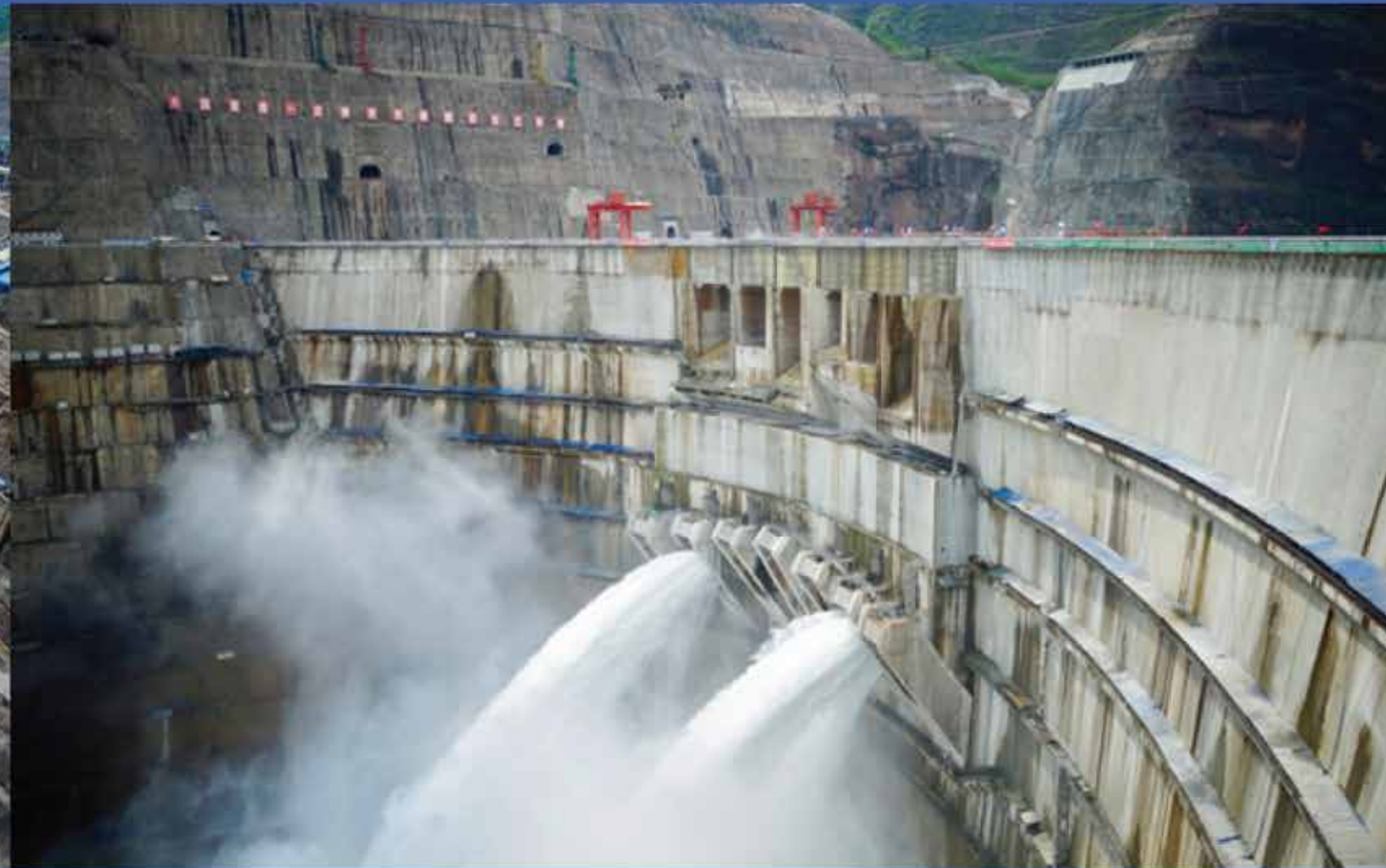
The Baihetan Dam opens to release water.
