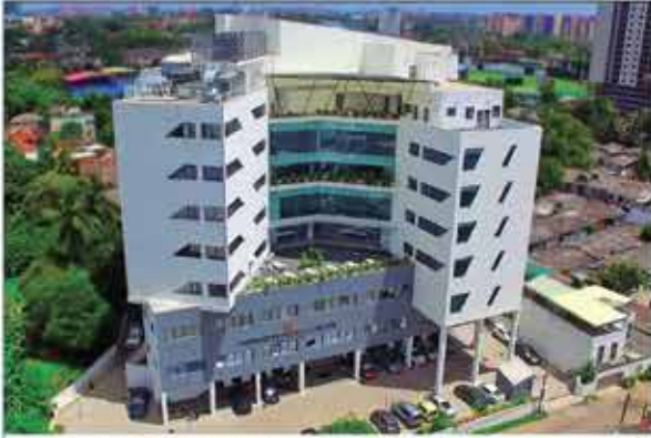
Rodney Street Development Project of Post Graduate Institute of Medicine, University of Colombo
