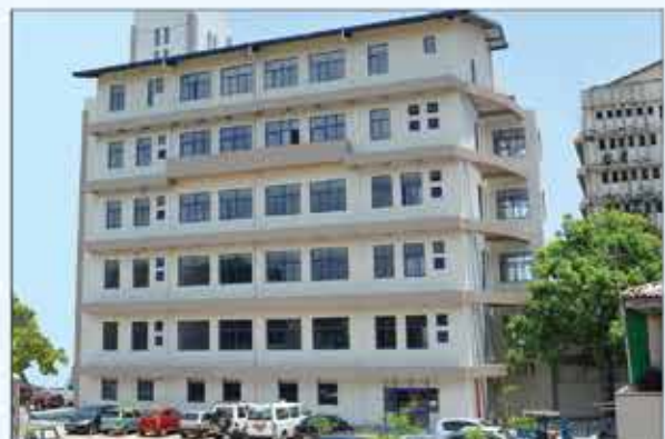
Construction of Police hospital Expansion Project in Narahenpita
