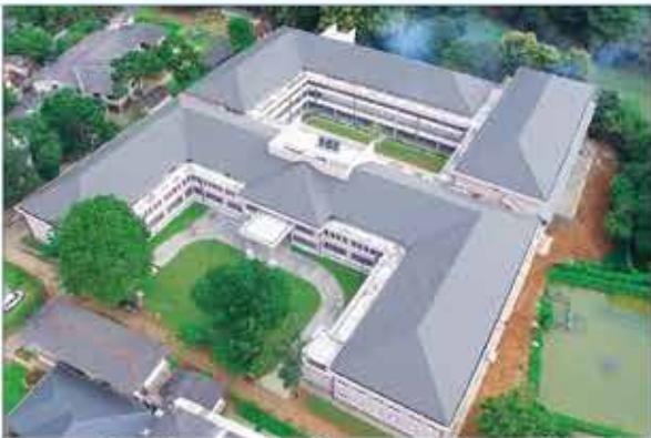
Design and Construction of Animal Science Building Complex, University of Peradeniya
